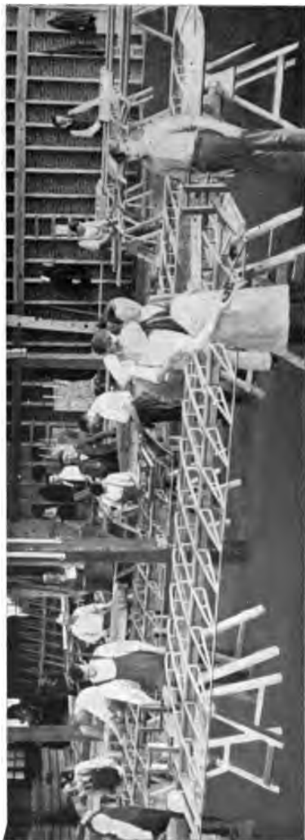
FIG. 132.—Building up the wings.
